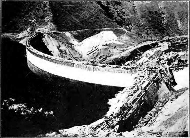
THE ARROW ROCK DAM (Idaho), still building in 1918 when this photo was taken: part of one of the most famous of all the government's projects to irrigate arid lands. This dam is 67 feet higher than the great Roosevelt Dam in Arizona.
